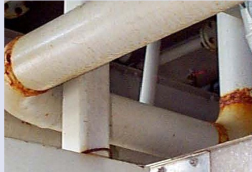
Weld / field joint coating failure
