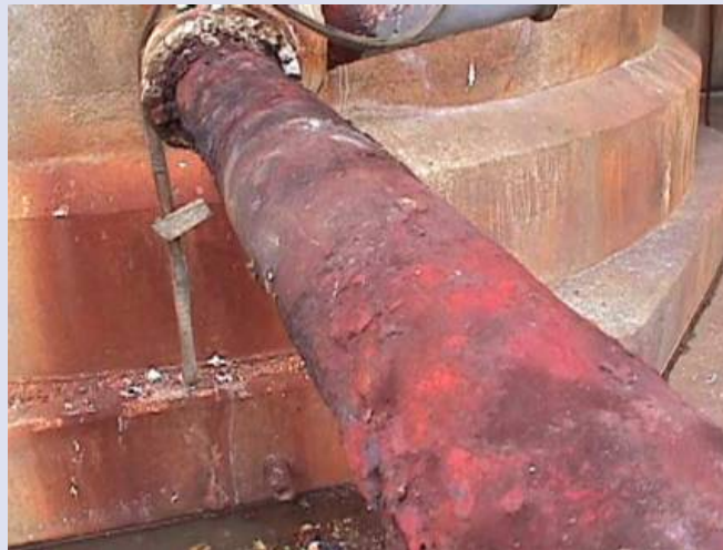
Corrosion under insulation
